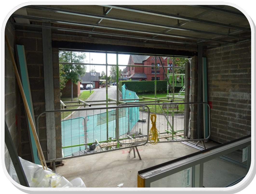
Looking out towards the care home from one of the apartments
