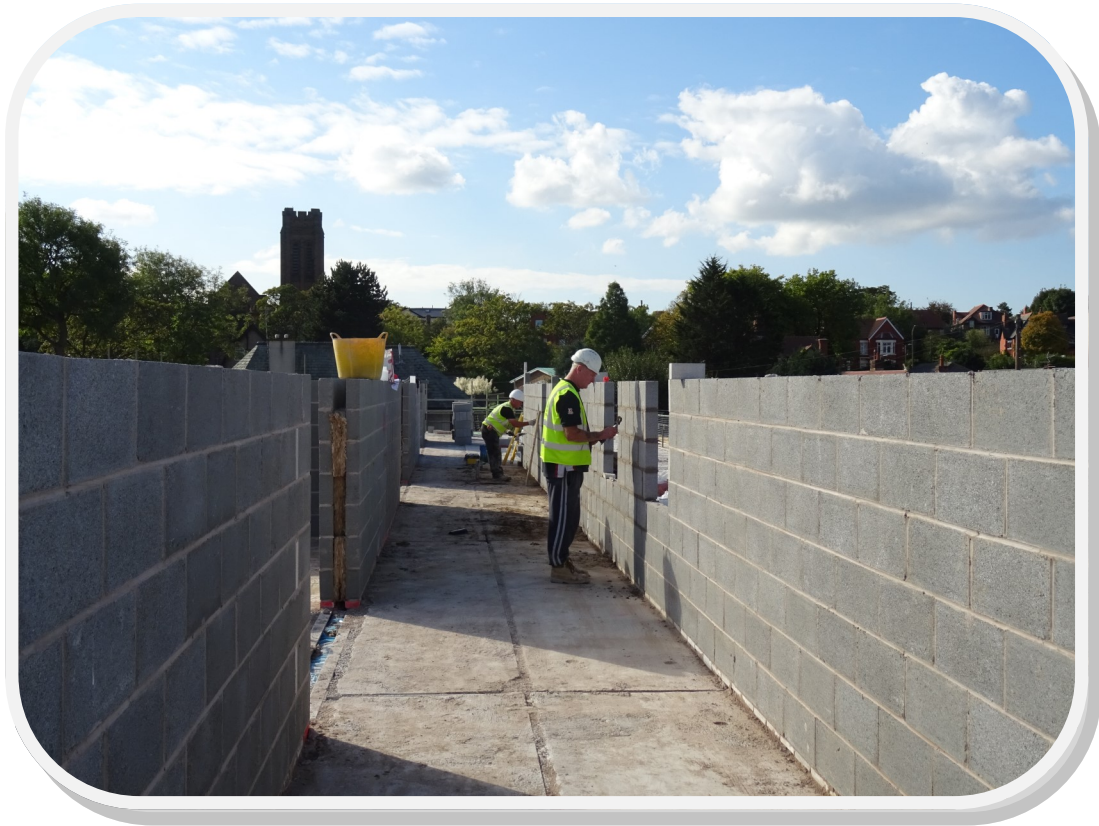
Internal brickwork being done up on the third floor
