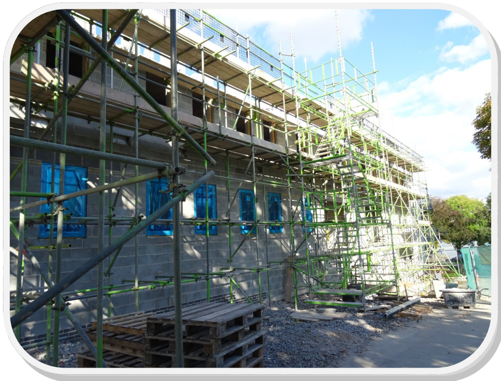
Windows starting to be put in on the first floor
