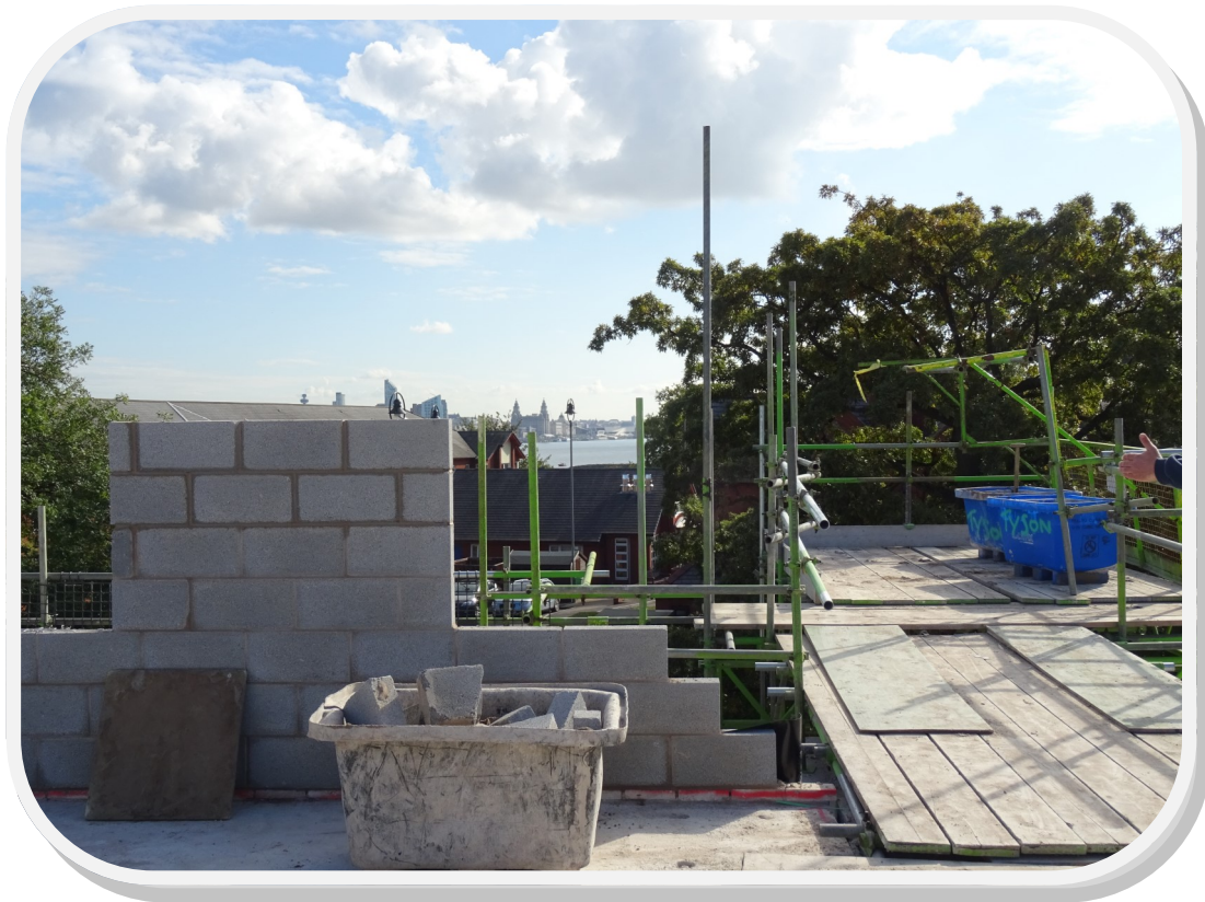
Looking towards the care home from the third floor
